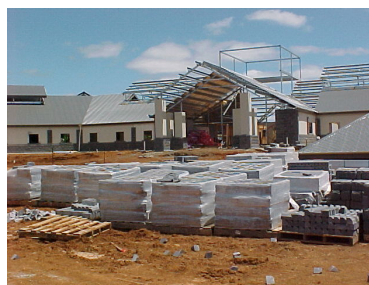
Equestrian Centre under construction
