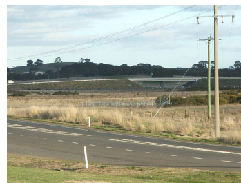
Calder Freeway bypass
