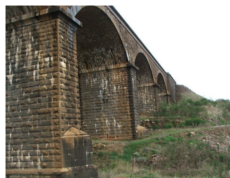
Bluestone railway viaduct
