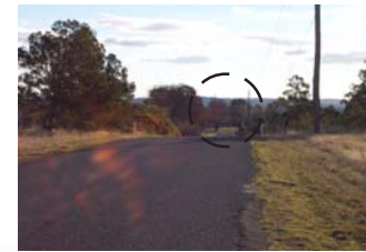
Existing Malmsbury East Road which will become the Melbourne entry to Malmsbury once the bypass is operational. Note the two affected Elms in the distance which could be relocated.
