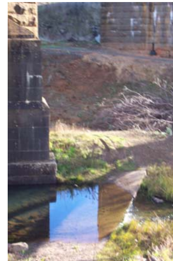
Existing crossing at Viaduct is inundated for most of the year
