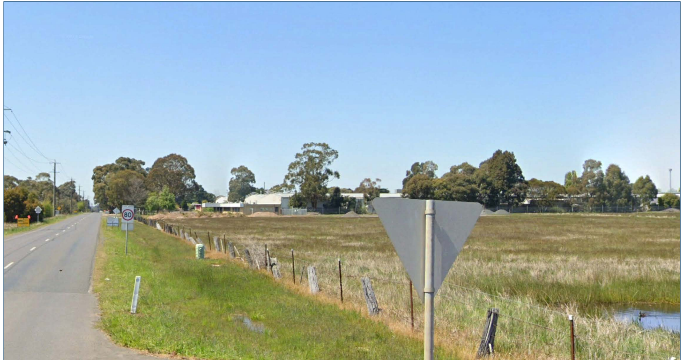
Corner of Hamilton and Barringo Roads, looking south-east. Image sourced from Google Streetview (October 2022) due to intersection upgrades at the time of the site visit.
