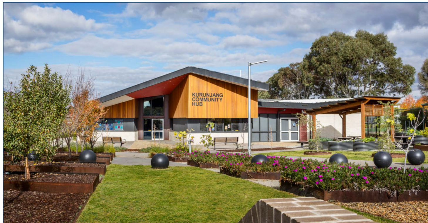
Example community centre in Melton which uses a combination of landscaping, architecture and materials to manage its visual appearance. (City of Melton and Brand Architects)
