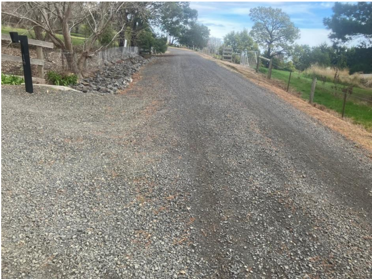
Figure 2 - Access Lane looking up hill
