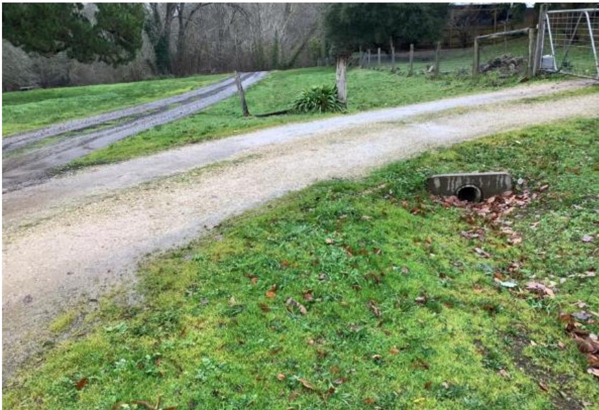
Figure 6 – Culvert draining from Pohlman Street
