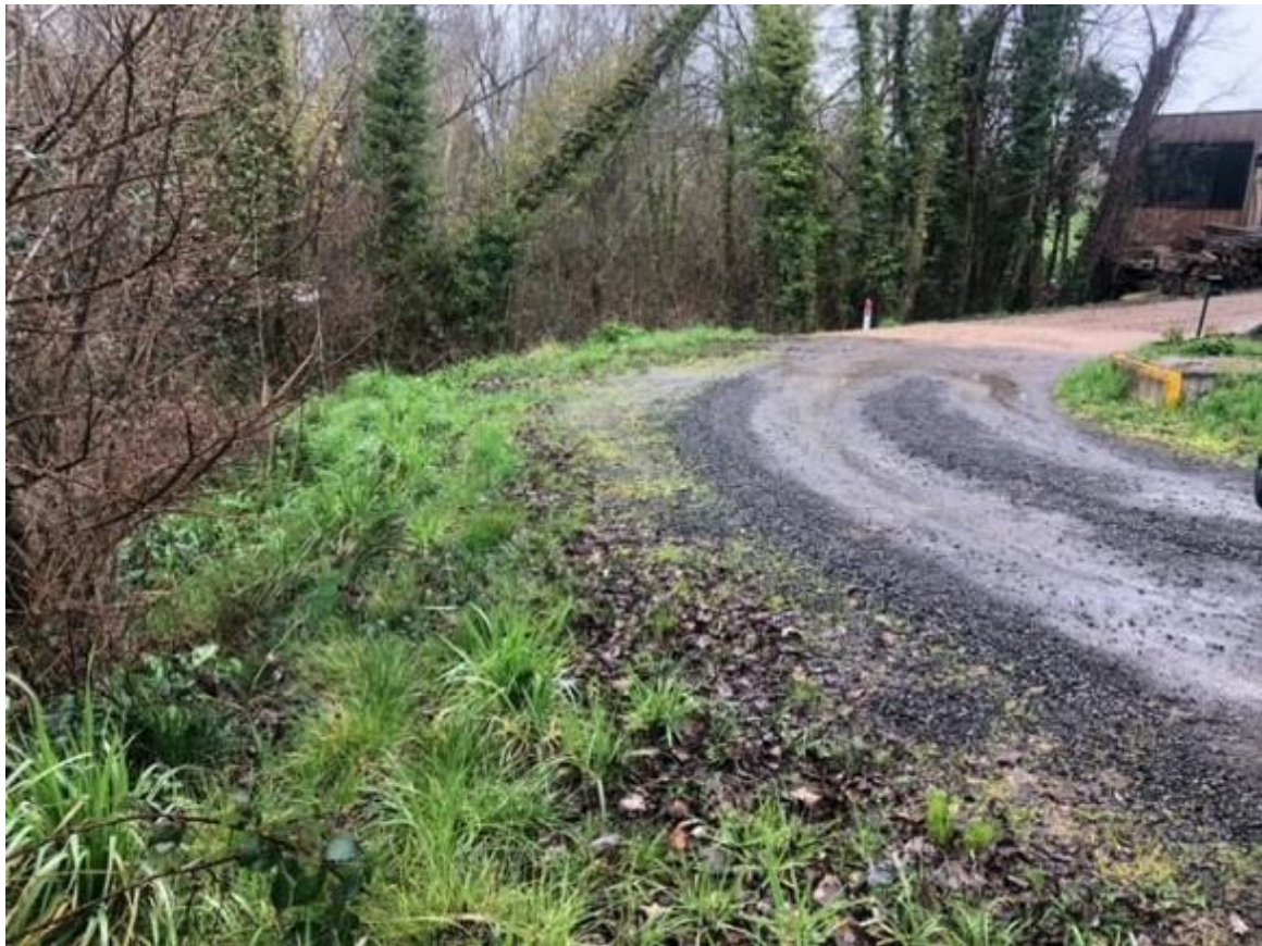
Figure 5 - Existing dead-end condition showing vegetation and drop
