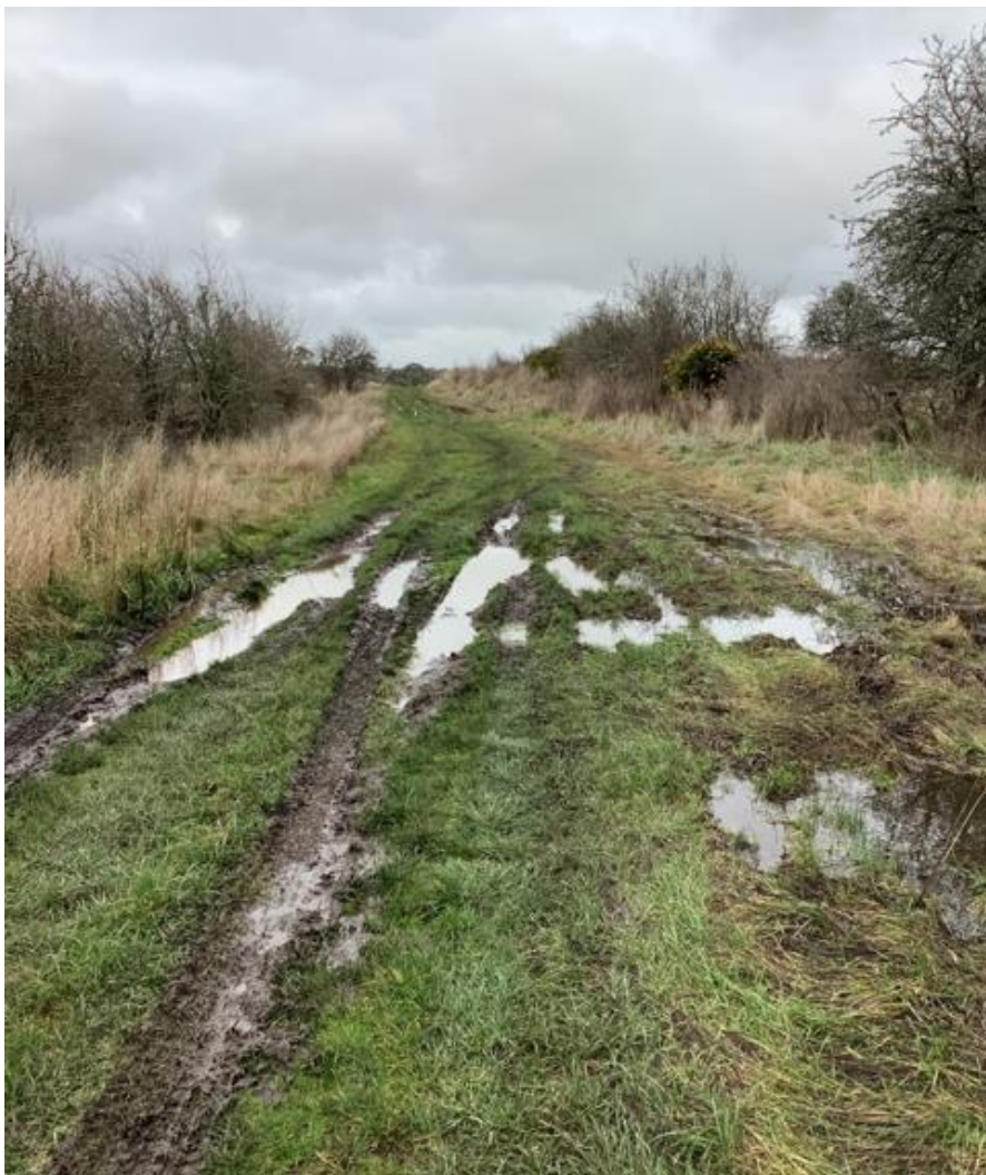
Figure 4 – Requested road section
