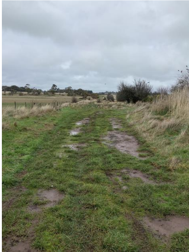
Figure 5 – Requested road section
