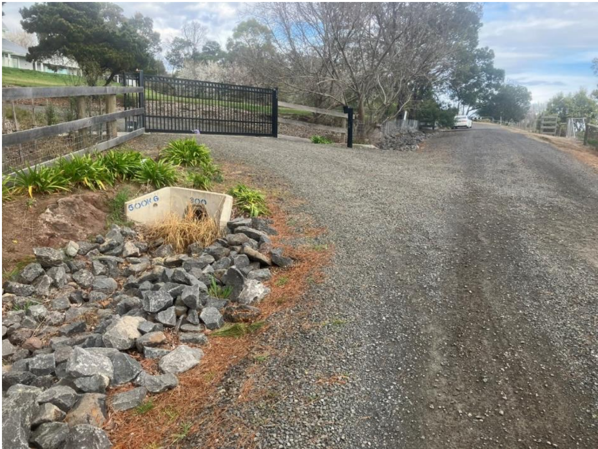
Figure 3 – Existing swale drain and culvert on crossing
