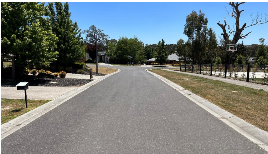
FIGURE 8: VIEW ON ECHIDNA LANE AT FAIRWAY DRIVE INTERSECTION (FACING NORTHWEST)
