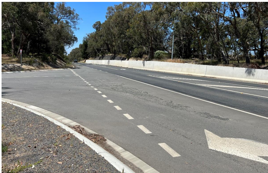
FIGURE 4: VIEW ON MELTON ROAD FACING NORTHEAST
