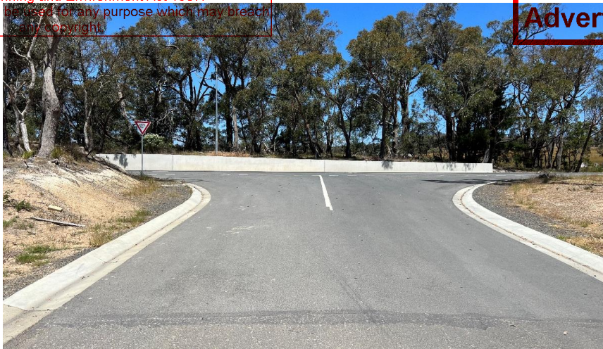
FIGURE 7: VIEW ON BIRDIE WAY AT MELTON ROAD INTERSECTION (FACING SOUTH)
