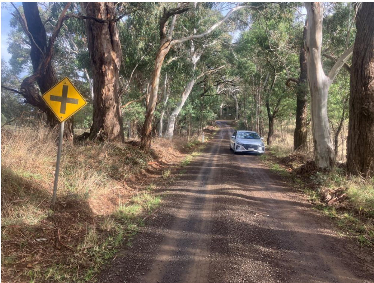
Figure 3 – Existing drainage system on Segment 1
