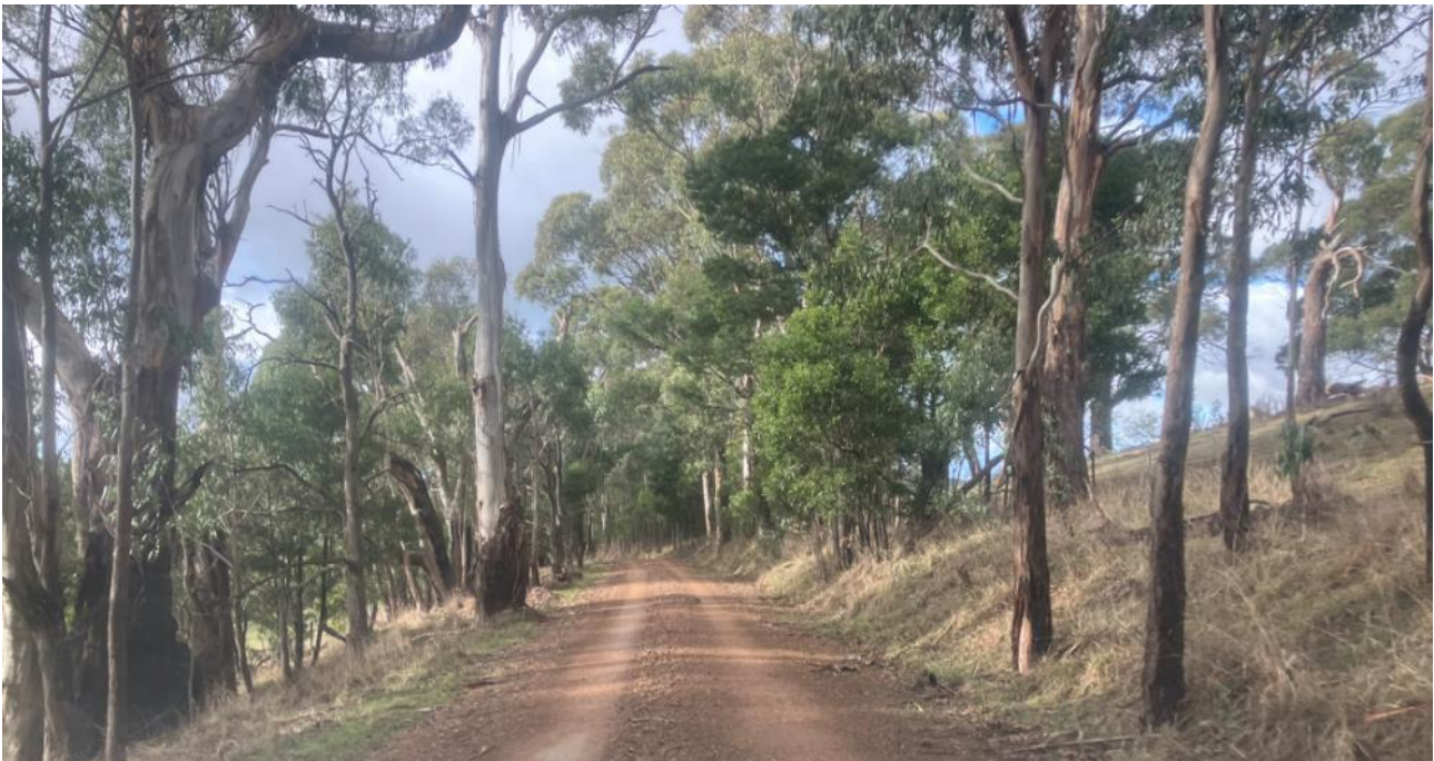
Figure 5 – Existing drainage condition on Segment 3.
