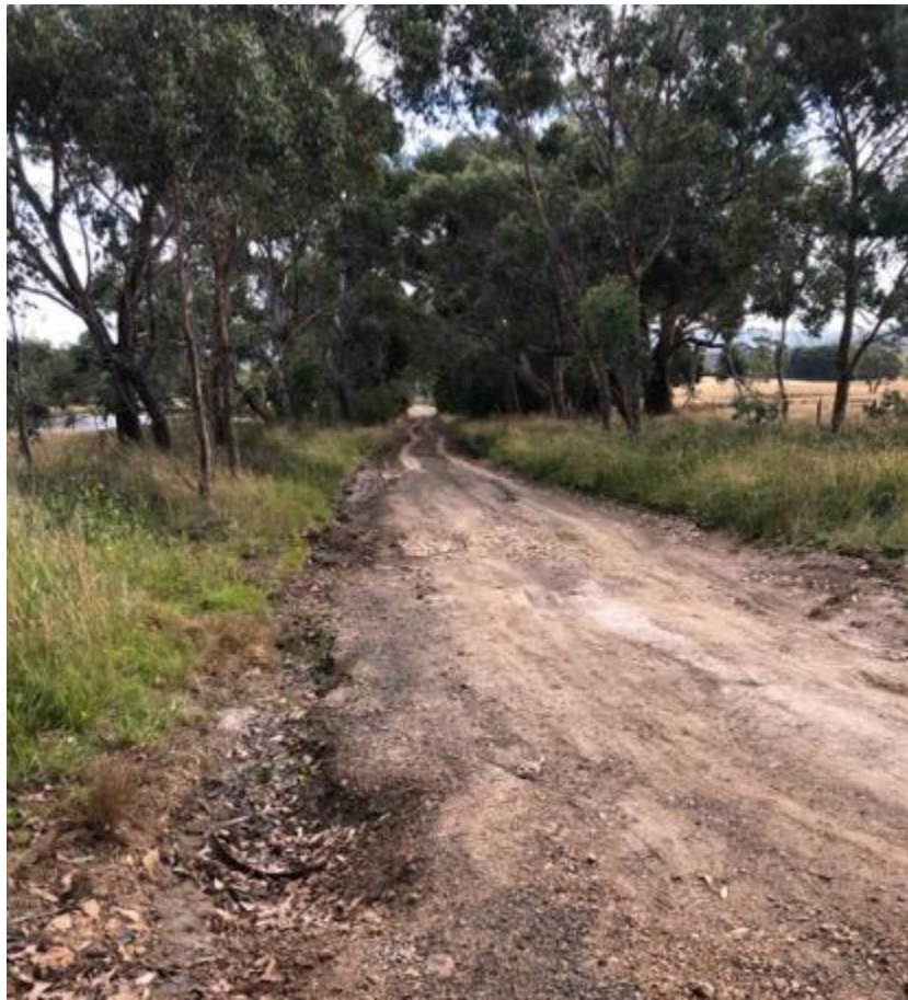
Figure 3 – East end of Pattinsons Lane requested section
