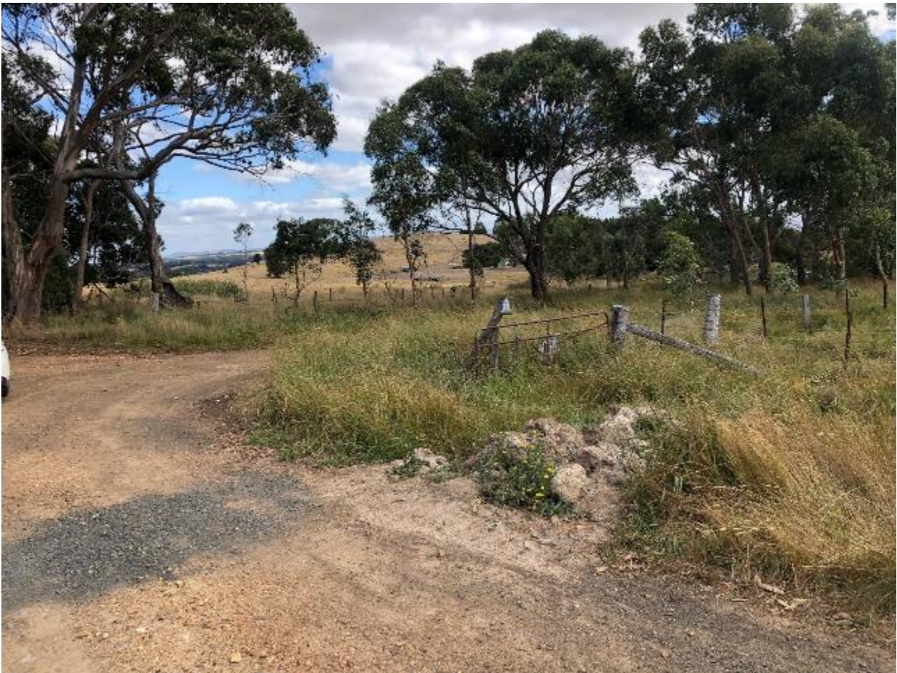
Figure 8 – Culvert draining from Fagans Ln to Patterson Lane
