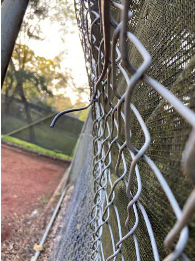
█ Courts 1&2. Protruding wire. Committee tries to thread these wires back in but as fences move these wires make their way back out. (2023).
