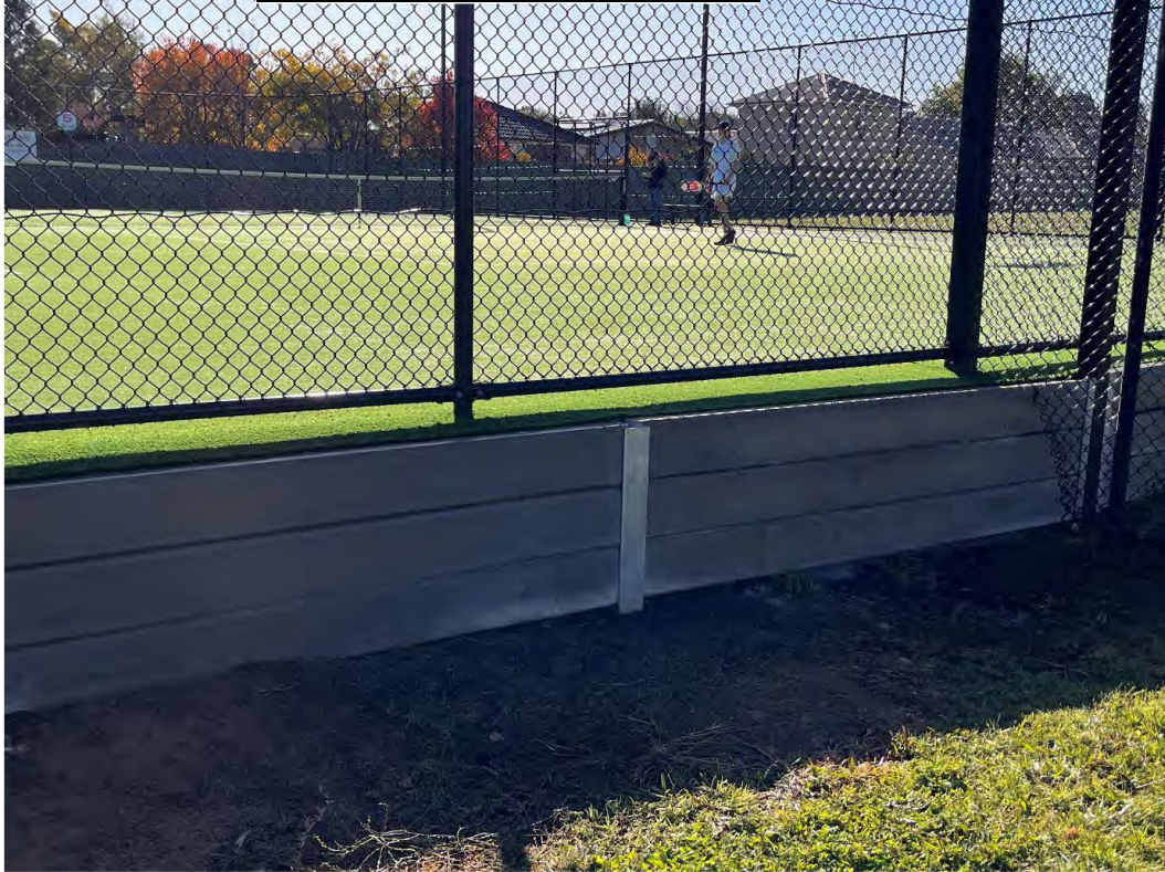
Example of concrete sleeper retaining wall with tennis fence integrated as required for courts 1-4. Retaining wall height will vary from 1 to 3 sleepers high at [REDACTED]. Image [REDACTED] (May 2023).
