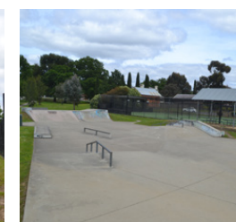
Skatepark overview facing south.
