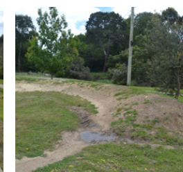
Eroded berm.
