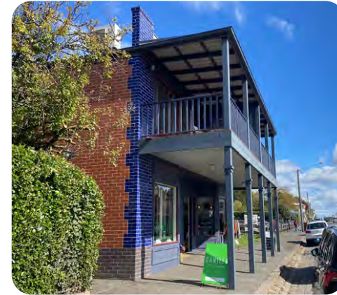
New development on Piper Street that is sympathetic to the heritage style without trying to mimic it
