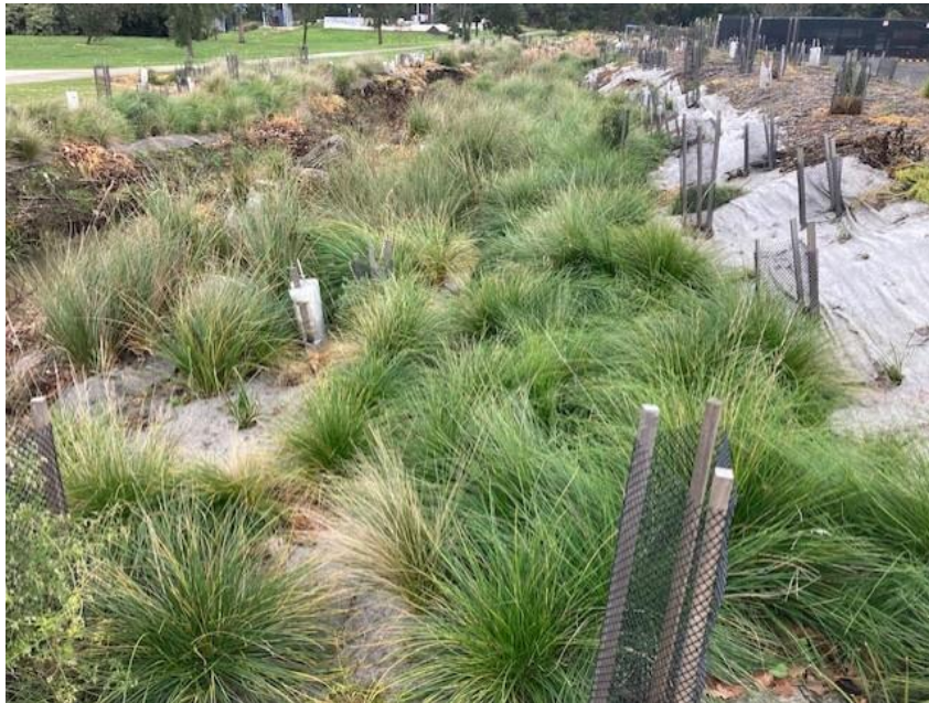
Bunjil Creek waterway restoration works, Gisborne
