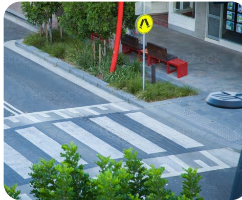
Kerb outstands create space for small public realm nodes that offer respite on a busy street and opportunities to incorporate WSUD into the town centre, like in Singleton NSW
