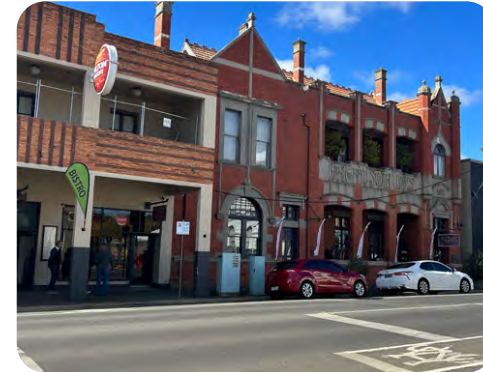
Heritage buildings along the main streets contribute greatly to the character of the town
