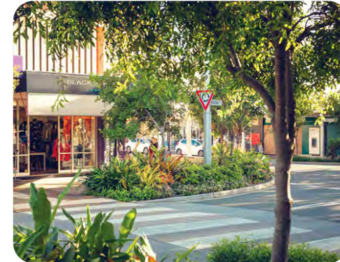
Planting and kerb outstands incorporated into crossings helps to narrow the carriageway, providing a shorter crossing distance and encouraging vehicles to slow down
