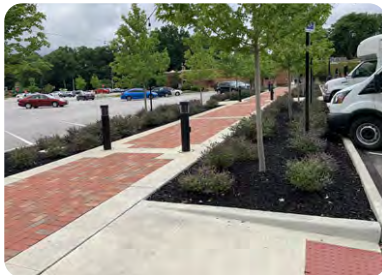
A clearly defined pedestrian pathway through a car park can increase safety and reduce points of conflict with cars
