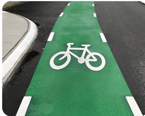
Marked cycle lanes provide a clear and consistent cycling route for streets with a higher volume of traffic, where sharrows are not appropriate
