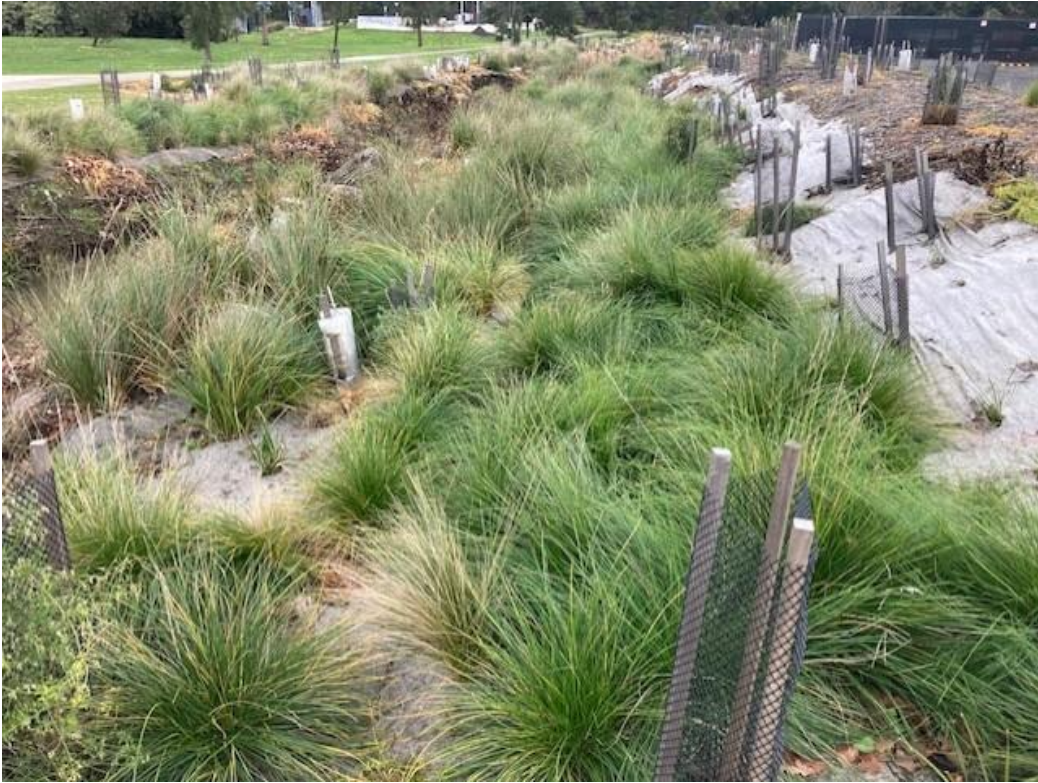
Bunjil Creek waterway restoration works, Gisborne
