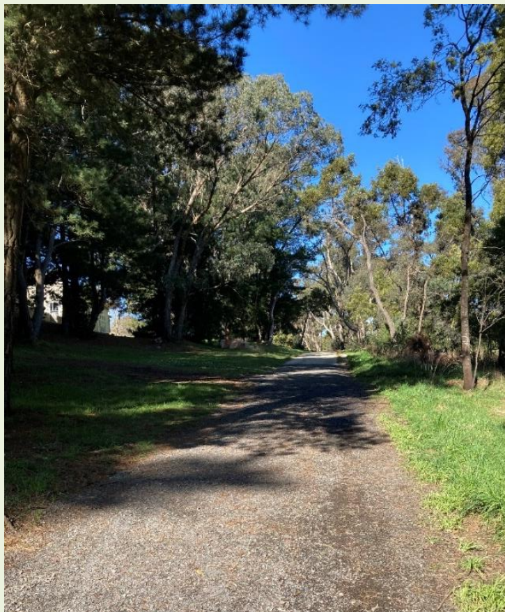
A constructed section of Stage 1A of the Macedon Ranges Shared Trail in Woodend
