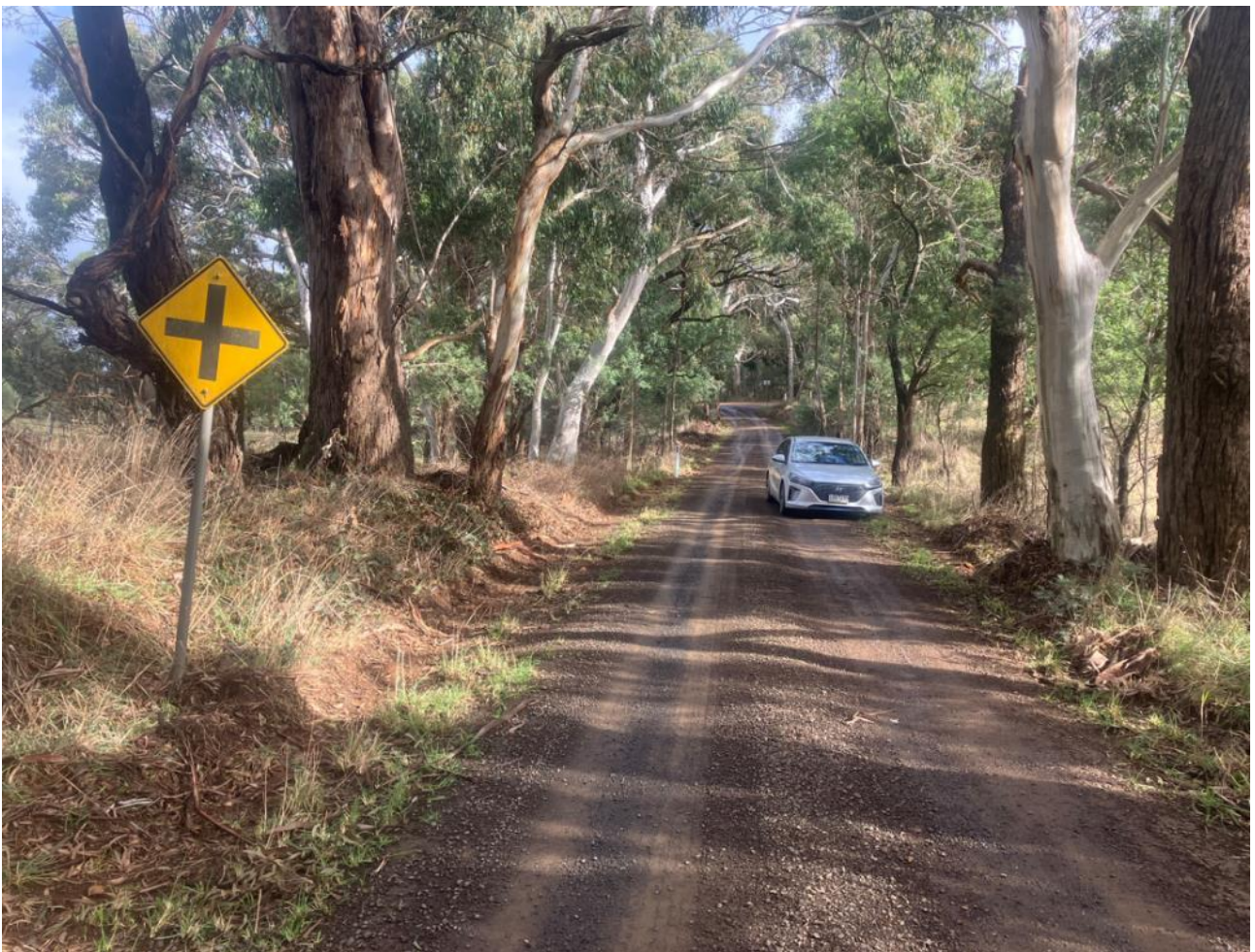
Figure 3 – Existing drainage system on Segment 1
