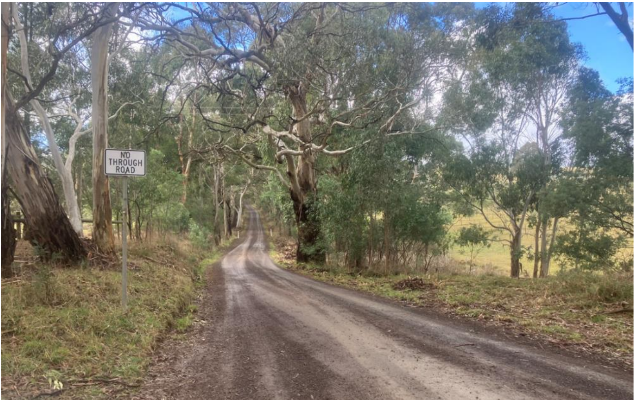
Figure 2 – Segment 1 near the West Goldie Rd intersection
