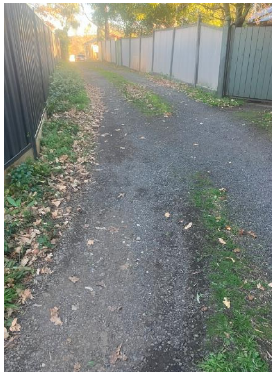
Figure 4 – Unmaintained Access Lane. Photo from the mid-block looking inwards.
