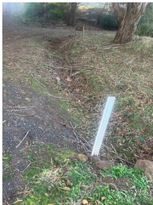
Figure 7 – Existing drainage system
