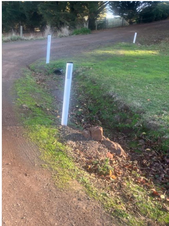
Figure 4 – Table drain near to the Bend of Magnet lane
