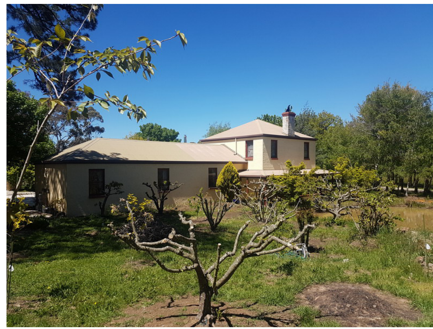
SUBJECT SITE: 286 CENTRAL ROAD TYLDEN EXISTING TWO STOREY RENDERED HOUSE
