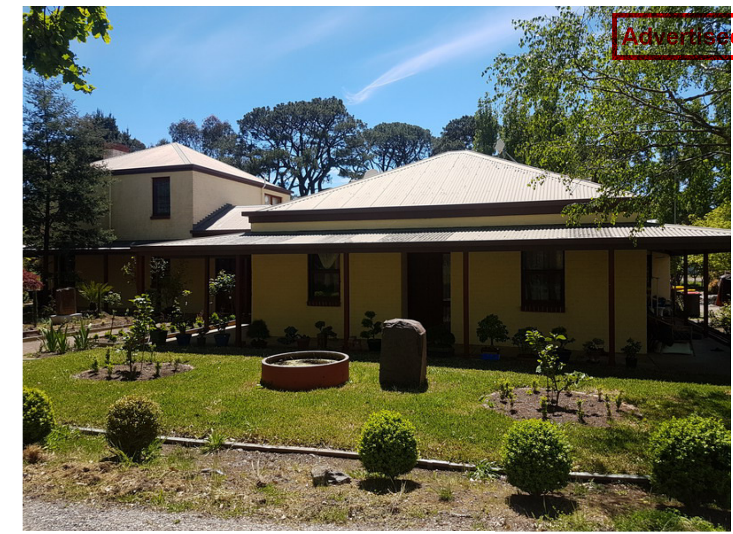
SUBJECT SITE: 286 CENTRAL ROAD TYLDEN EXISTING TWO STOREY RENDERED HOUSE
