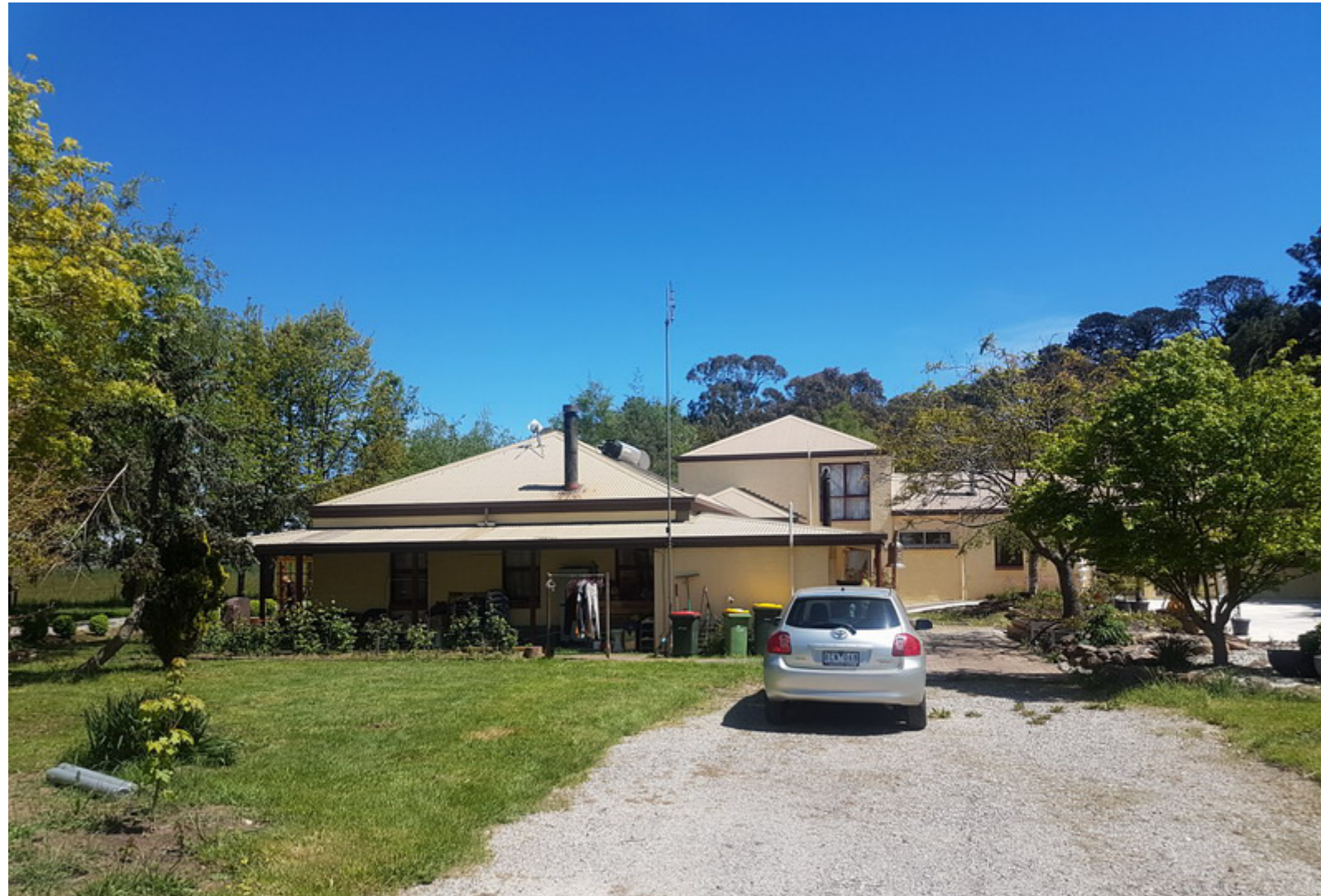
SUBJECT SITE: 286 CENTRAL ROAD TYLDEN EXISTING TWO STOREY RENDERED HOUSE
