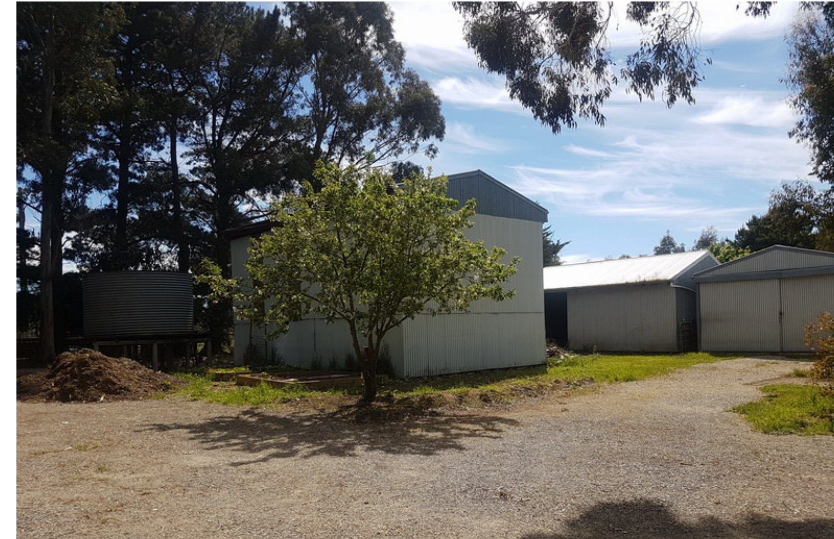
SUBJECT SITE: 286 CENTRAL ROAD TYLDEN EXISTING SHEDS
