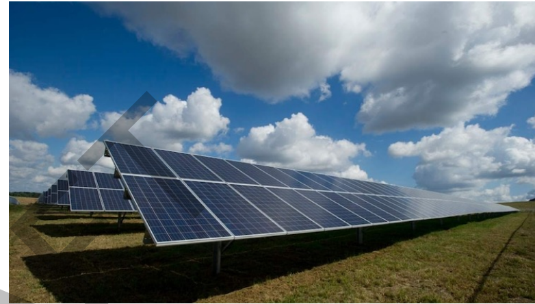
Victoria's biggest solar farm under construction amid debate over lost agricultural land - ABC News
