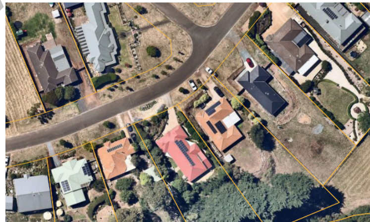
Rooftop solar in Romsey today (source Nearmap)
