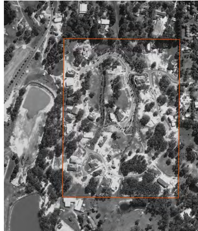
Figure 2. Dalton Street Precinct in 2010, under construction
