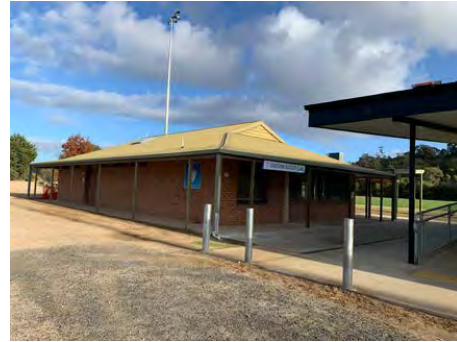
Gisborne Soccer club rooms
