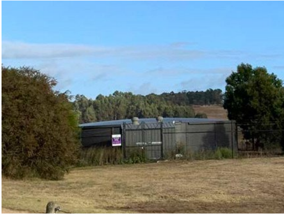
Water tank next to Croquet Club
