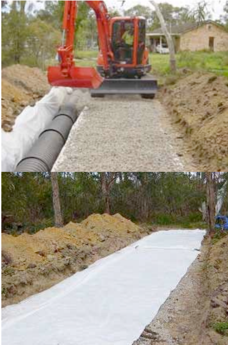
Figure 4 Backfilling gravel layer. Figure 5 Adding the second geotextile fabric layer
