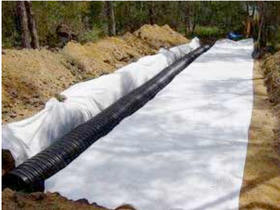
Figure 10.3 Laying the liner in the trench and then the geotextile fabric as the ‘wick’ across the pan
