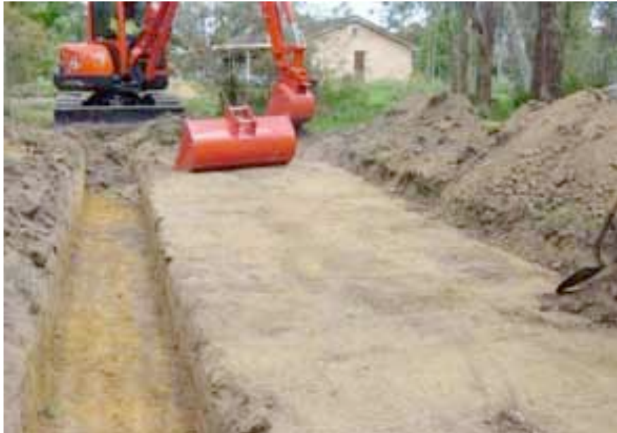
Figure 2 Excavation of the bed of the “Wick” trench
