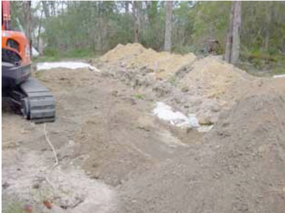
Figure 5 Backfilling and the inspection ports
